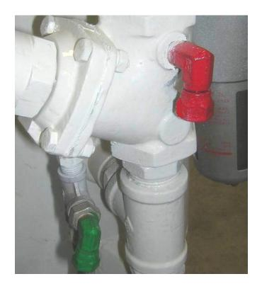
Connect the twin-line deadman hoses to the 1/8" BSP (green hose to green elbow) and 1/4 BSP (red hose to red elbow) swivel connections on the control valve.
