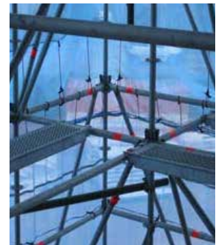
NOTE THE INCREASED NUMBER OF TIES AT THE CORNERS.
